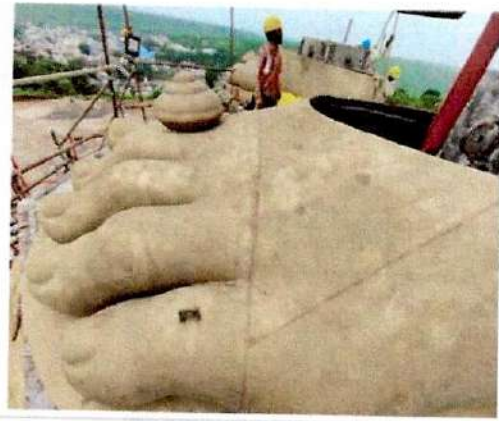
Bronze Panel Feet Erection
