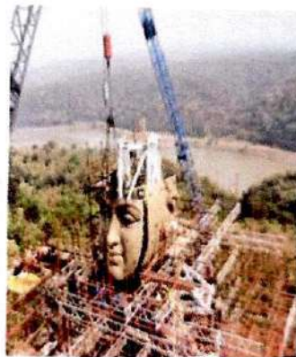
Bronze Panel Face Erection
