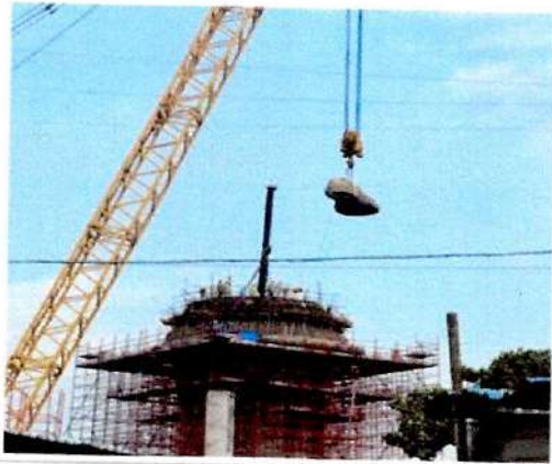
Bronze Panel Feet Erection
